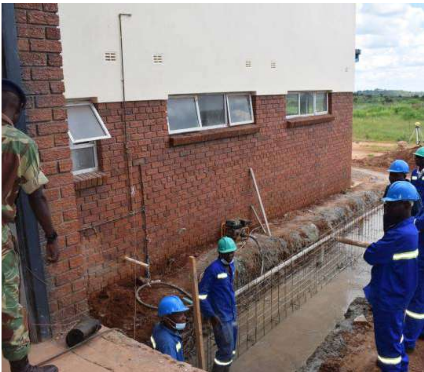
Construction of the Disused Radioactive Sources Management Facility proceeded well in 2022
