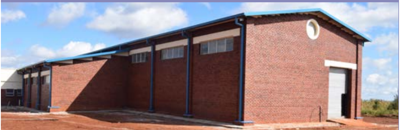
The Facility will receive, process and store disused radioactive sources, medical waste and other radioactive waste from industry and research.
