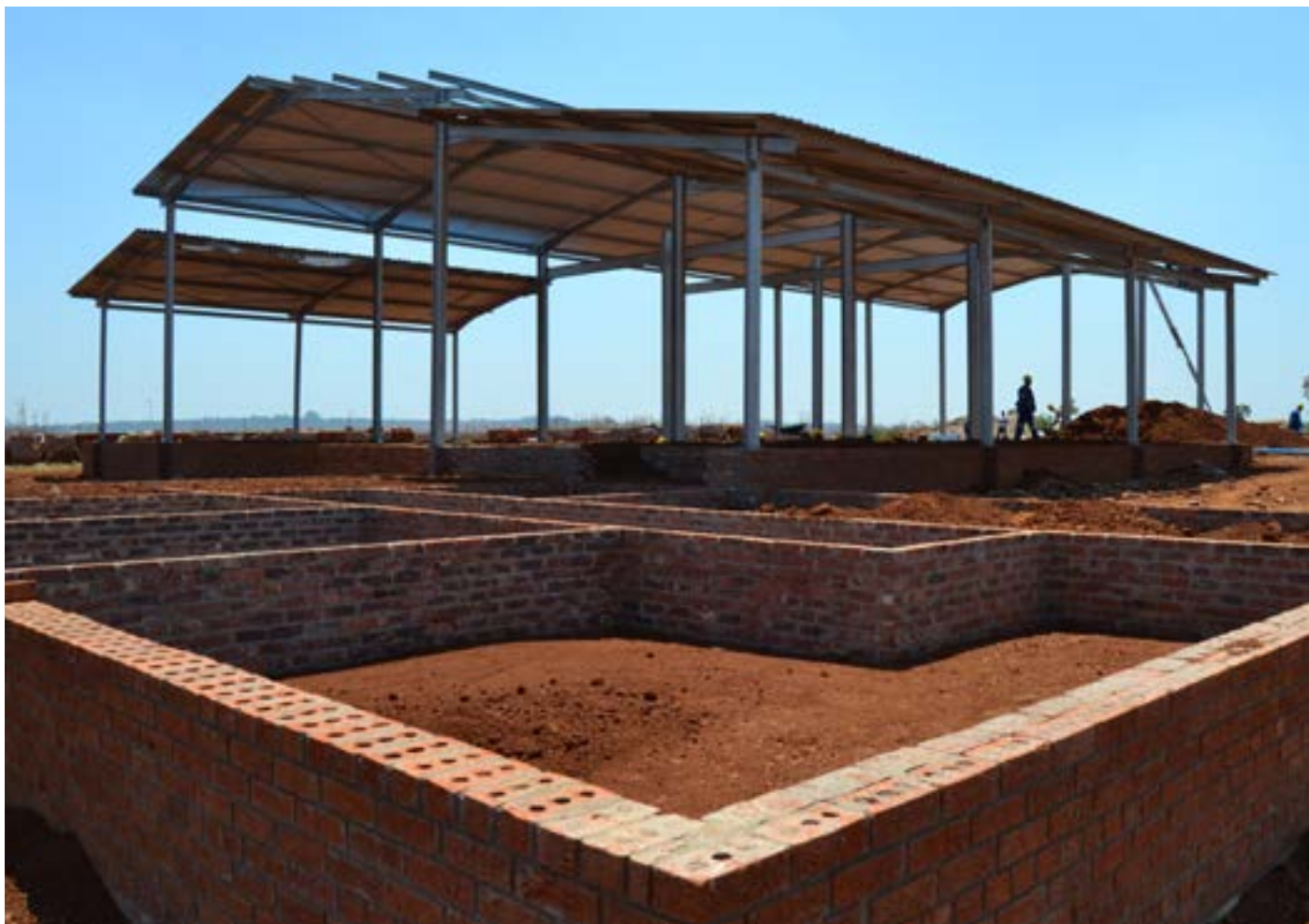
Construction works at the Disused Radioactive Sources Management Facility commenced in 2016.
